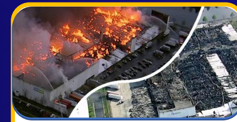
Thermal Fire Prevention
