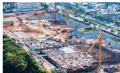
Construction Sites: "Keep Out"
